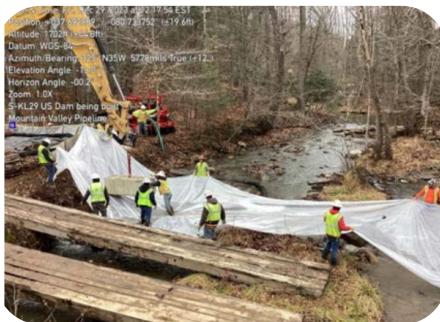
Constructing upstream dam.
