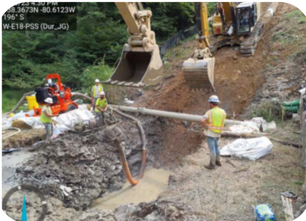
Contractor dewatering ditch line and ditching.
