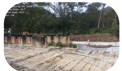
Timber Mats placed at Wetland (W-K333)
