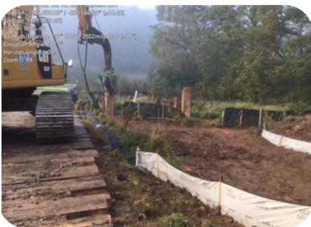
The sheet piling at W-K33.
