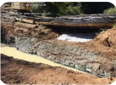
The excavation continued until pipe could be placed into crossing.
