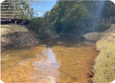
Downstream view of permitted impact area during post-construction assessment.
