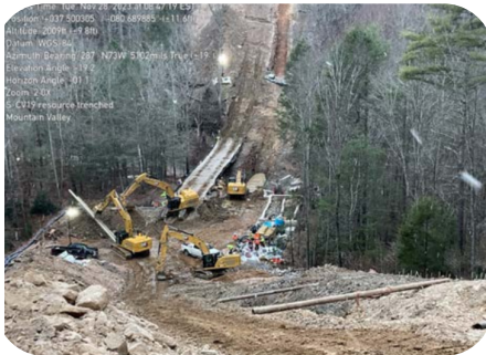
Excavating trench through aquatic resource.
