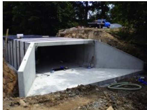
Precast box culvert installation. Photo credit: precast.org
