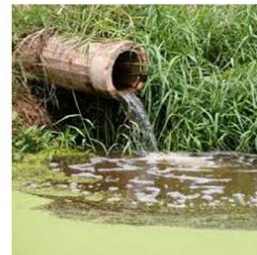
Pipe Discharging into Stream
