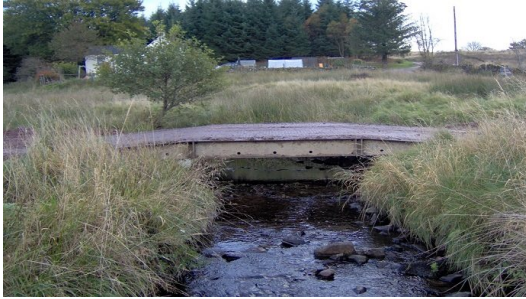
Temporary access bridge. Photo credit: mabeyhire.co.uk
