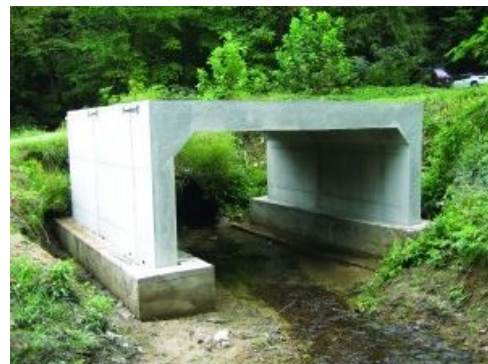
Bottomless box culvert installation. Photo credit: precast.org
