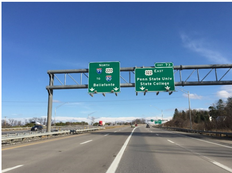
Arterial highway or expressway.
