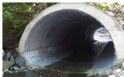
Pipe arch culvert. Photo credit: structuralguide.com/culvert
