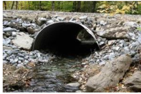
Open-bottomed arch culvert. Photo credit: co.ozaukee.wi.us
