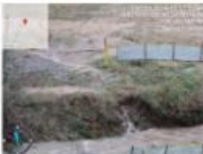
Sediment Laden Water Entering Stream
