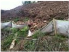
Failed Erosion Control
