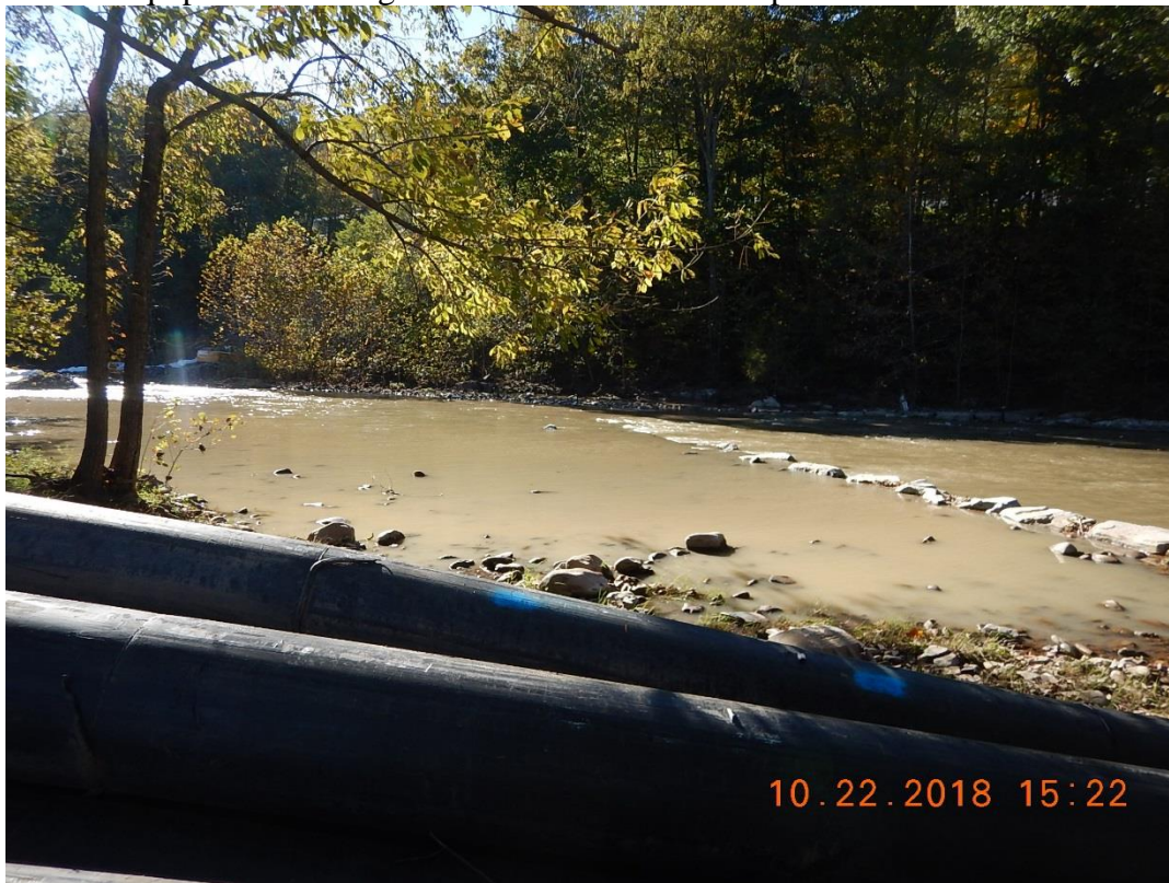
CNA and sediment laden water noted between the upstream dam and the discharge lines.
