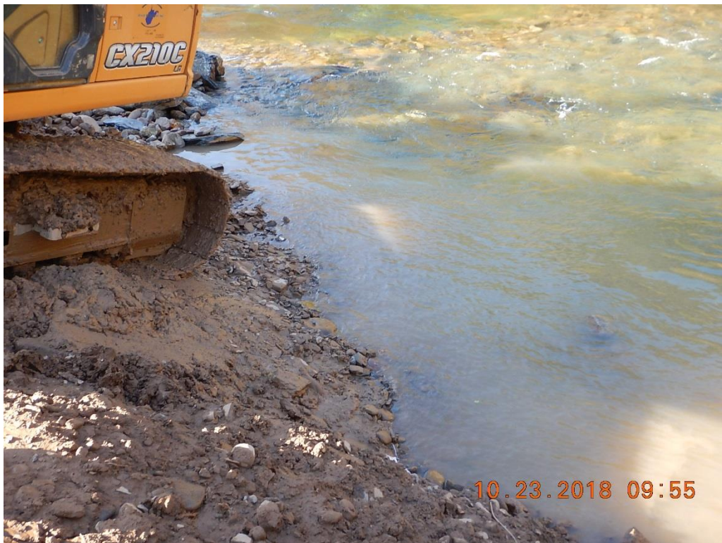
Equipment finishing pipe installation. Water still turbid.
