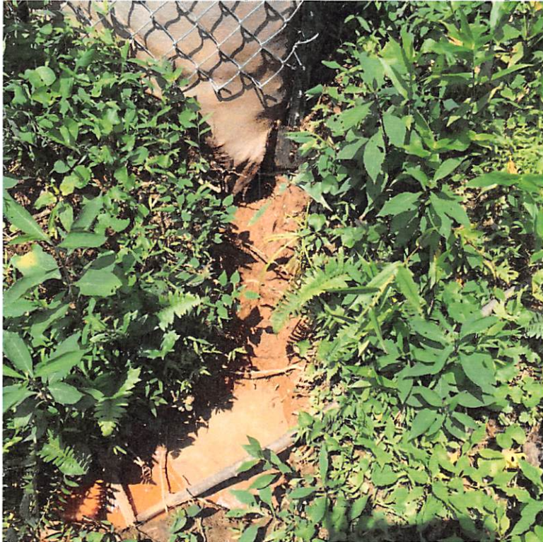
Sediment laden water leaving site at UNT of Jockey Camp Run due to concentrated flow damaging controls.
