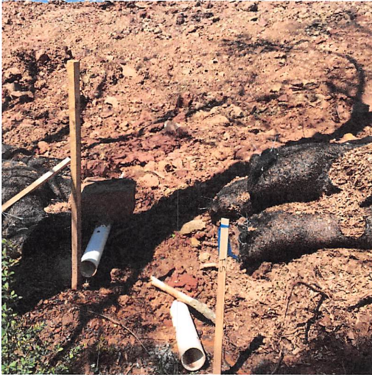
Improperly installed controls (removal of section of filter sock) at Sherwood Compressor.
