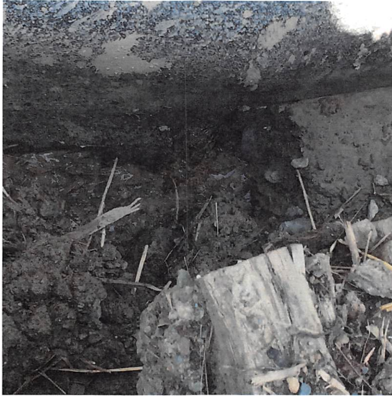
Hole in filter fabric at UNT of Nutter Fork causing sediment laden water to leave site.
