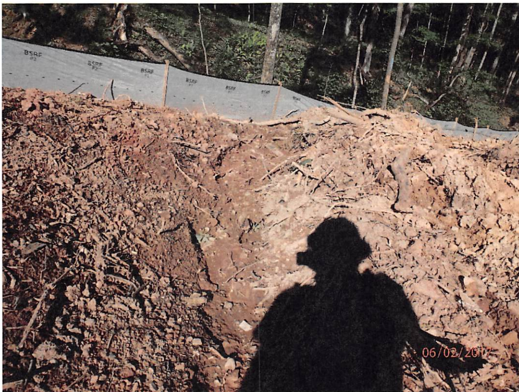
Concentrated flow from water bar that is following silt fence trench to the bottom of the hill near Rock Run.
