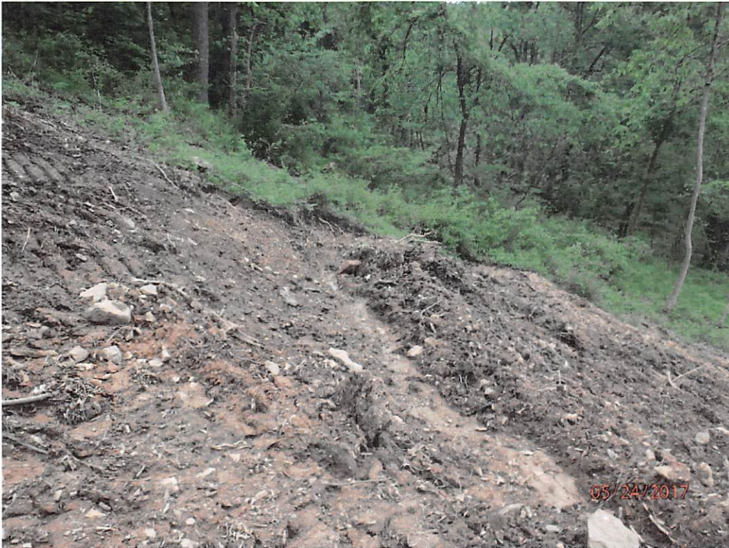
Water bar outlets that have no treatment, which is causing sediment laden water to leave site. The above pictures are representative of all water bars for the portion of the pipeline inspected.
