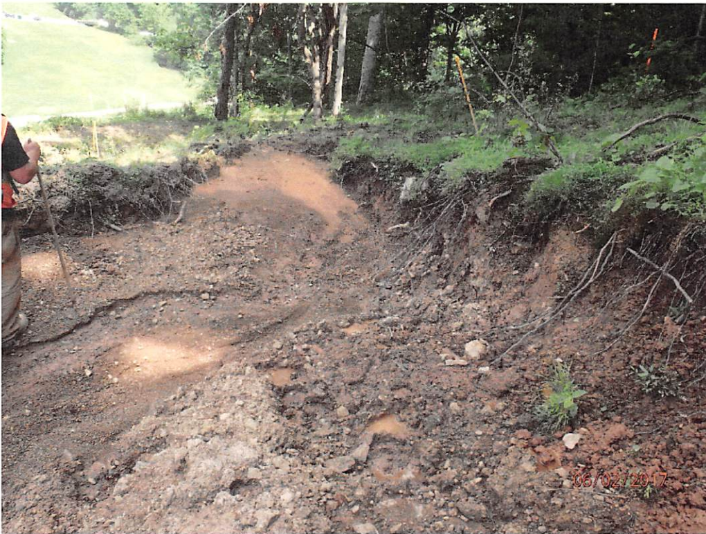
Water bar with no treatment at outlets.
