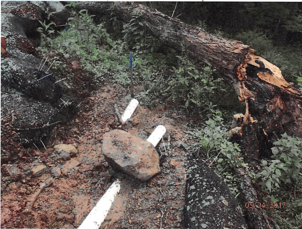
Portion of filter sock downslope of compressor site near Eibscamp Run that is improperly installed.
