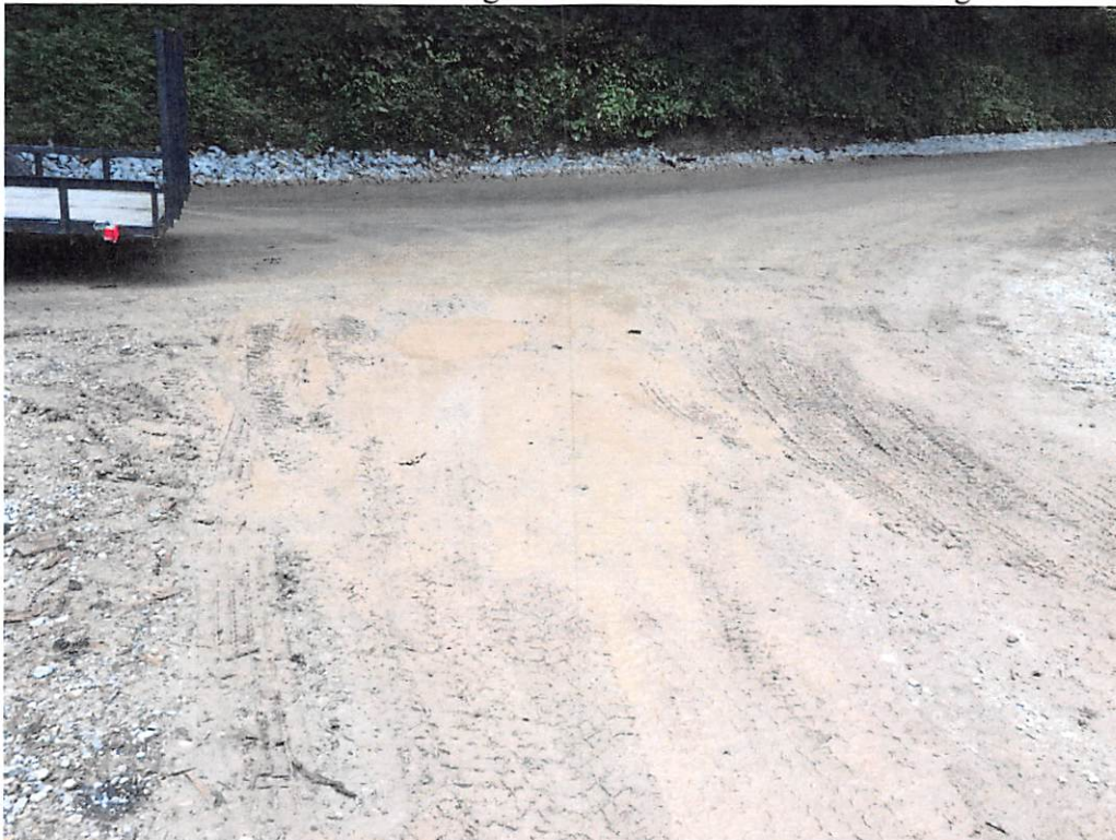
Unstable construction entrance causing mud to be tracked out onto Morgan's Run Road.
