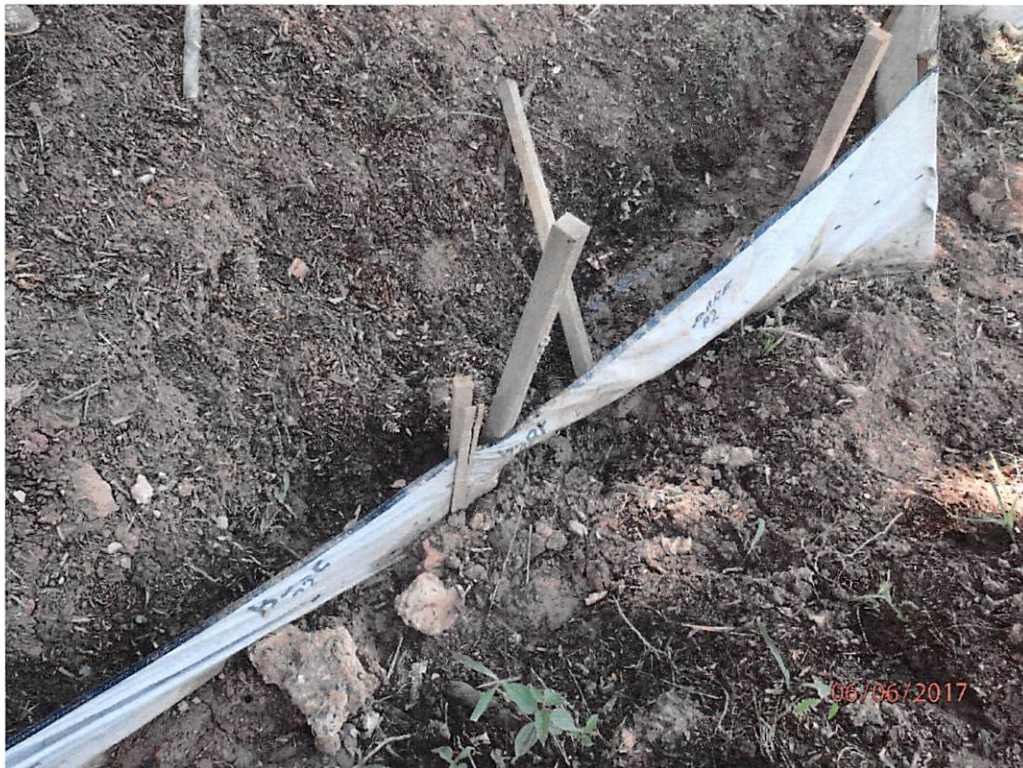
Improperly installed controls.
