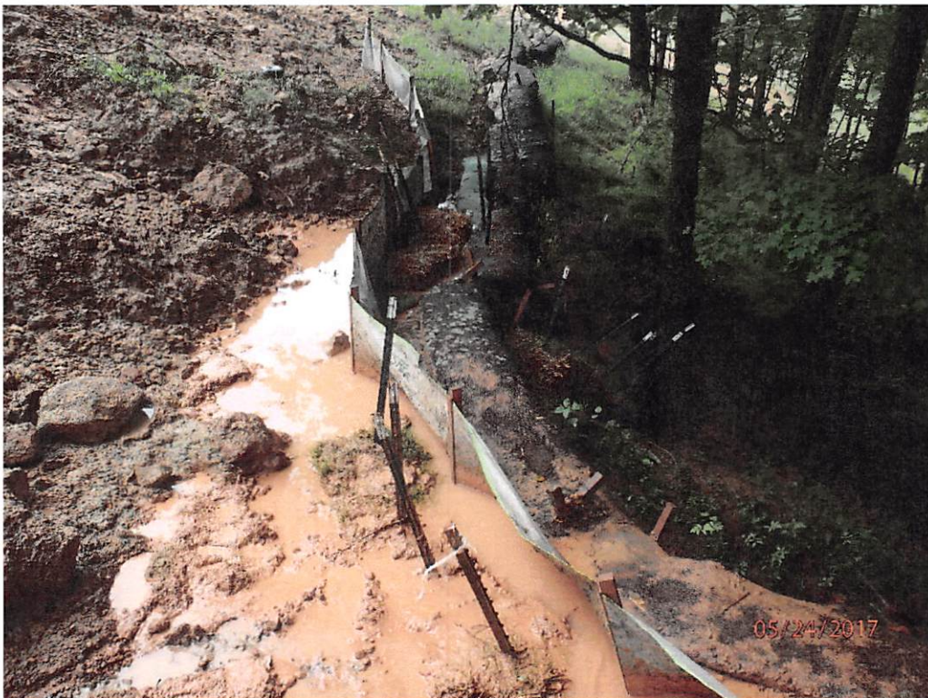
Area below compressor access road where concentrated flow is being treated with sheet flow controls. This area is consistently being overwhelmed which is causing sediment laden water to leave the site.
