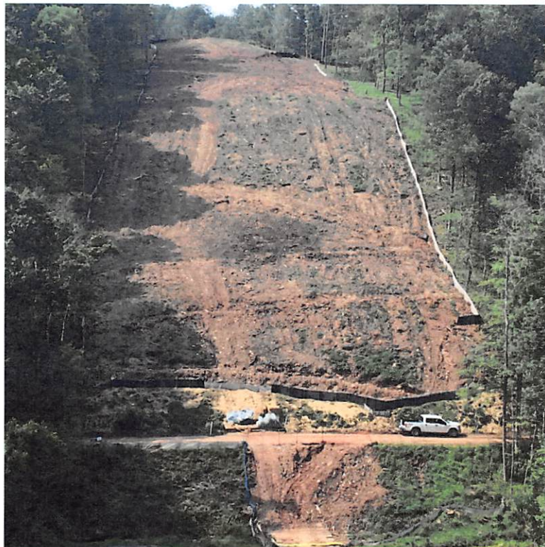
Area near Camp Mistake where water bars end prior to exiting perimeter silt fence.
