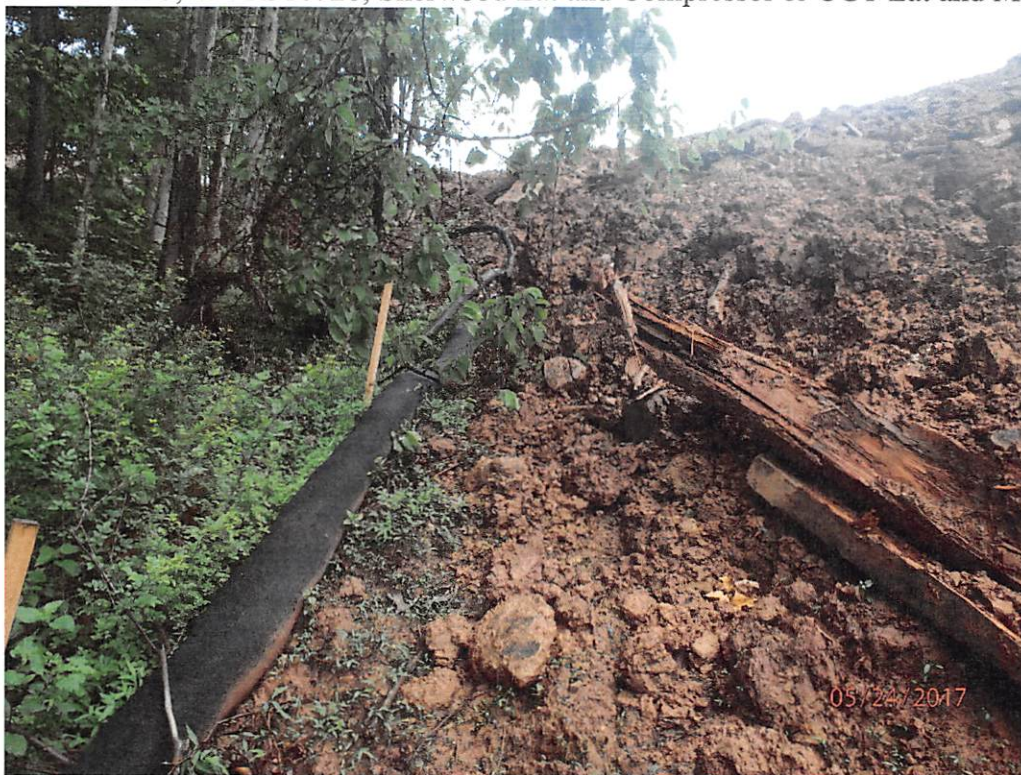
Area below access road near compressor site where construction activity has gone past LOD and compromised controls.
