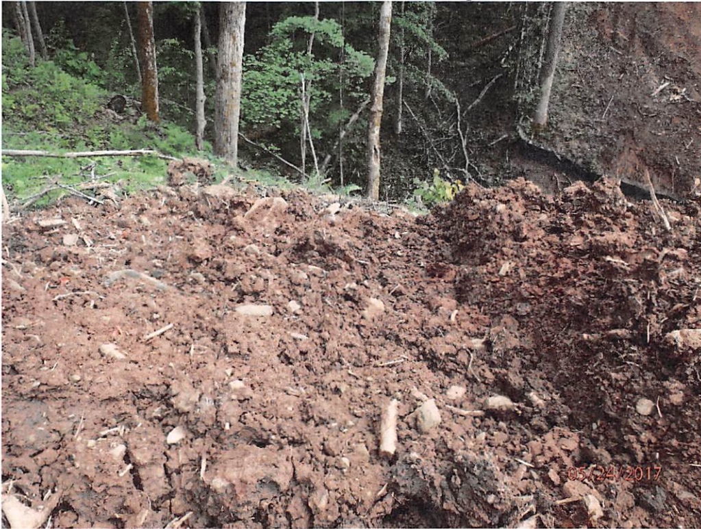
Water bar outlets that have no treatment, which is causing sediment laden water to leave site.
