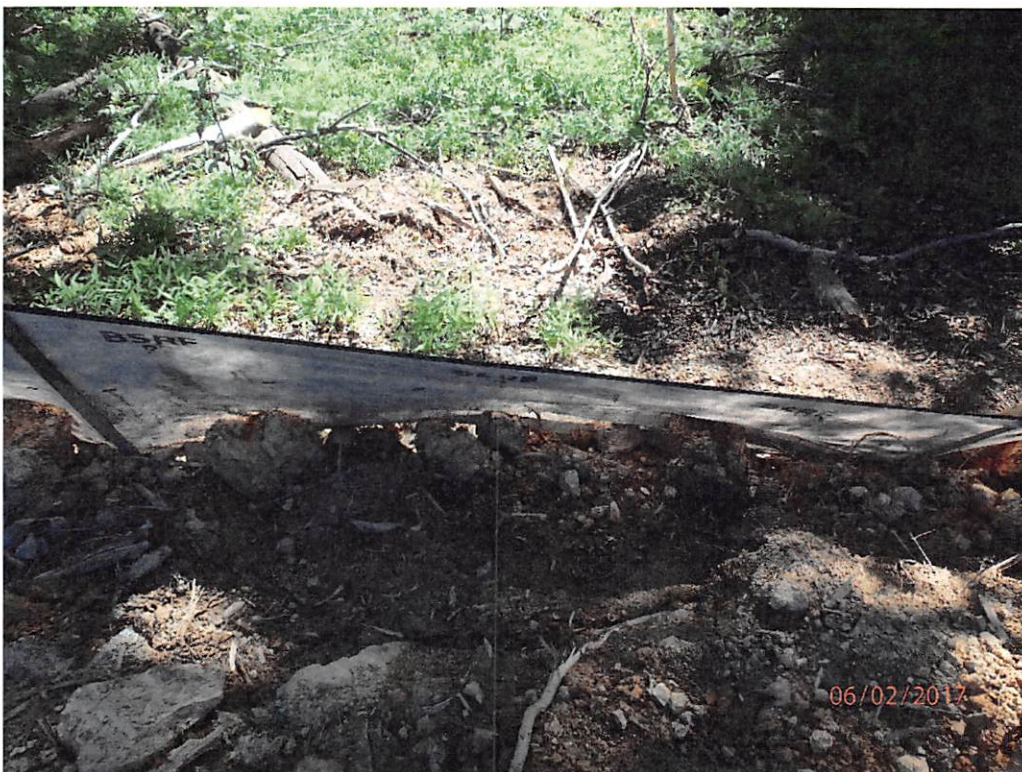
Improperly installed controls.
