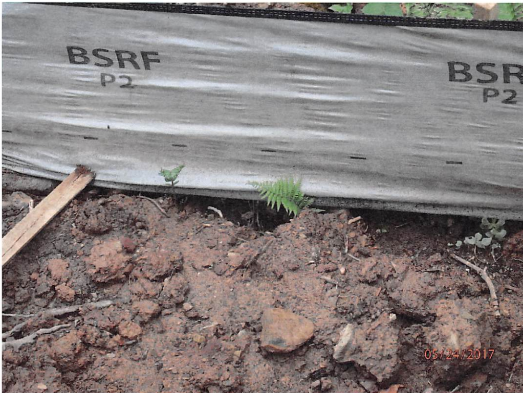
Improperly installed controls on Sherwood Lateral pipeline. Bottom picture is at stream crossing of UNT of Buckeye Creek.
