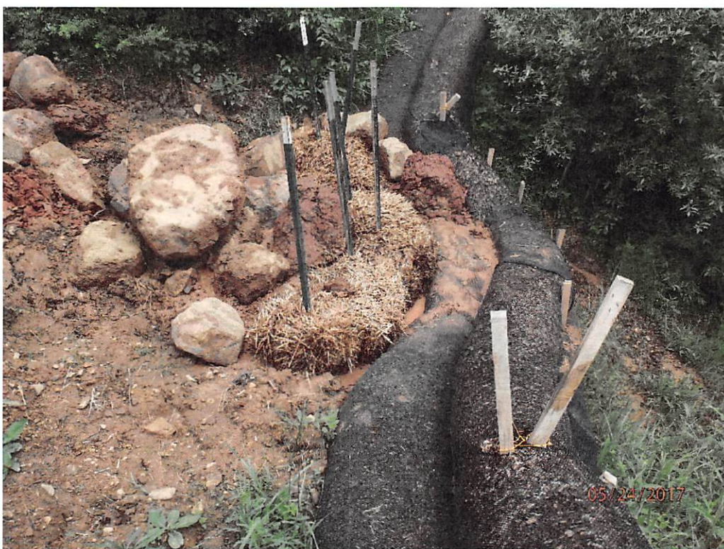
Perimeter controls below compressor site near Eibscamp Run.
