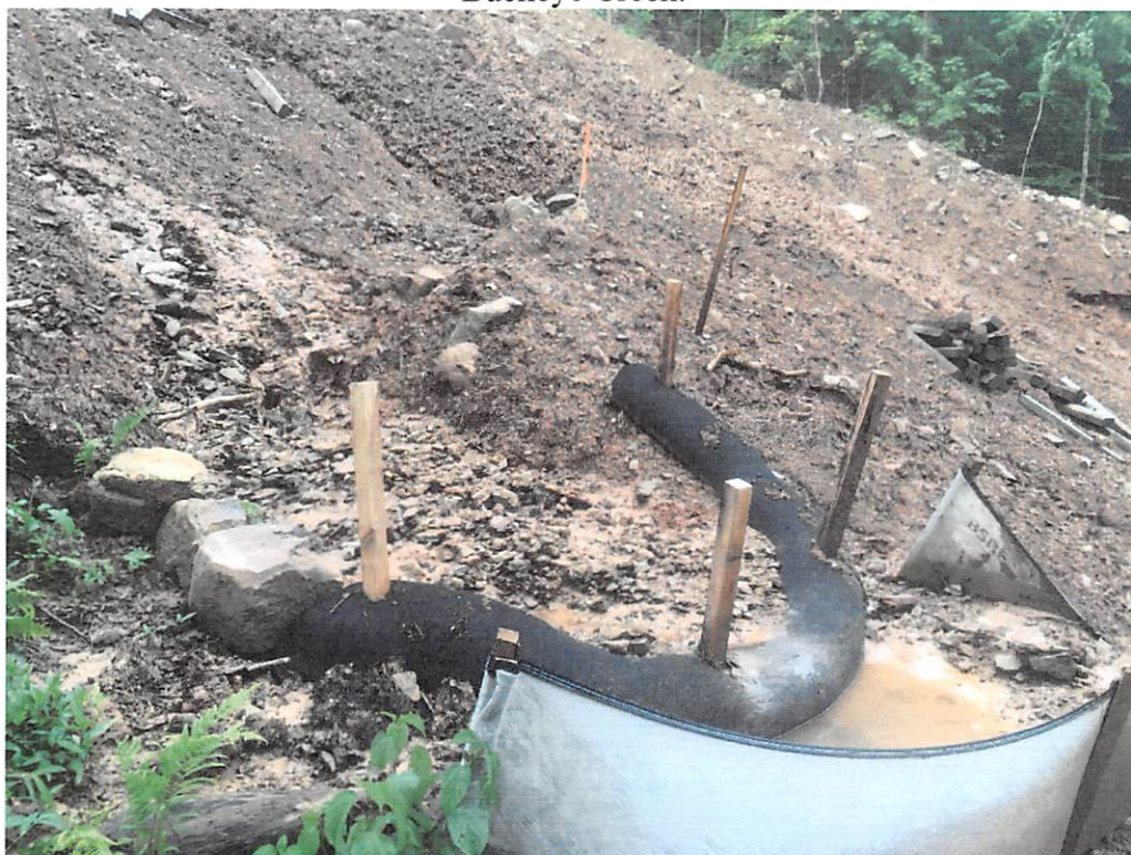
BMPs in need of maintenance near UNT of Buckeye Creek.
