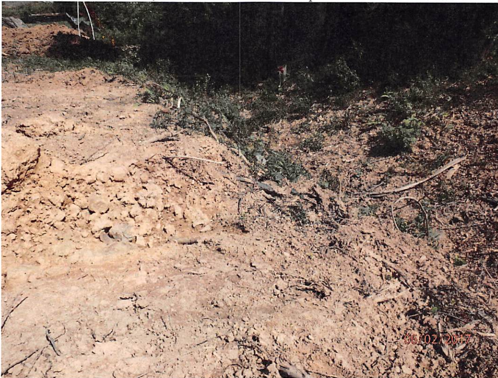
Water bar outlet that goes into ephemeral stream that leads off site with no controls in place.
