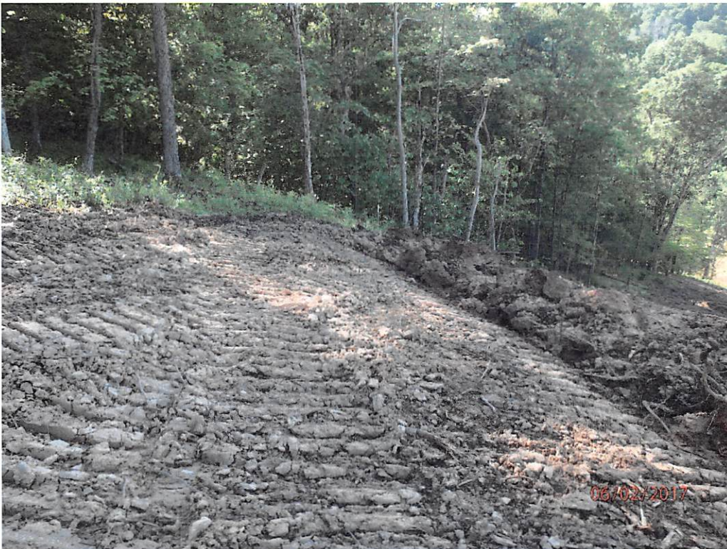
Water bars with no treatment at outlets.
