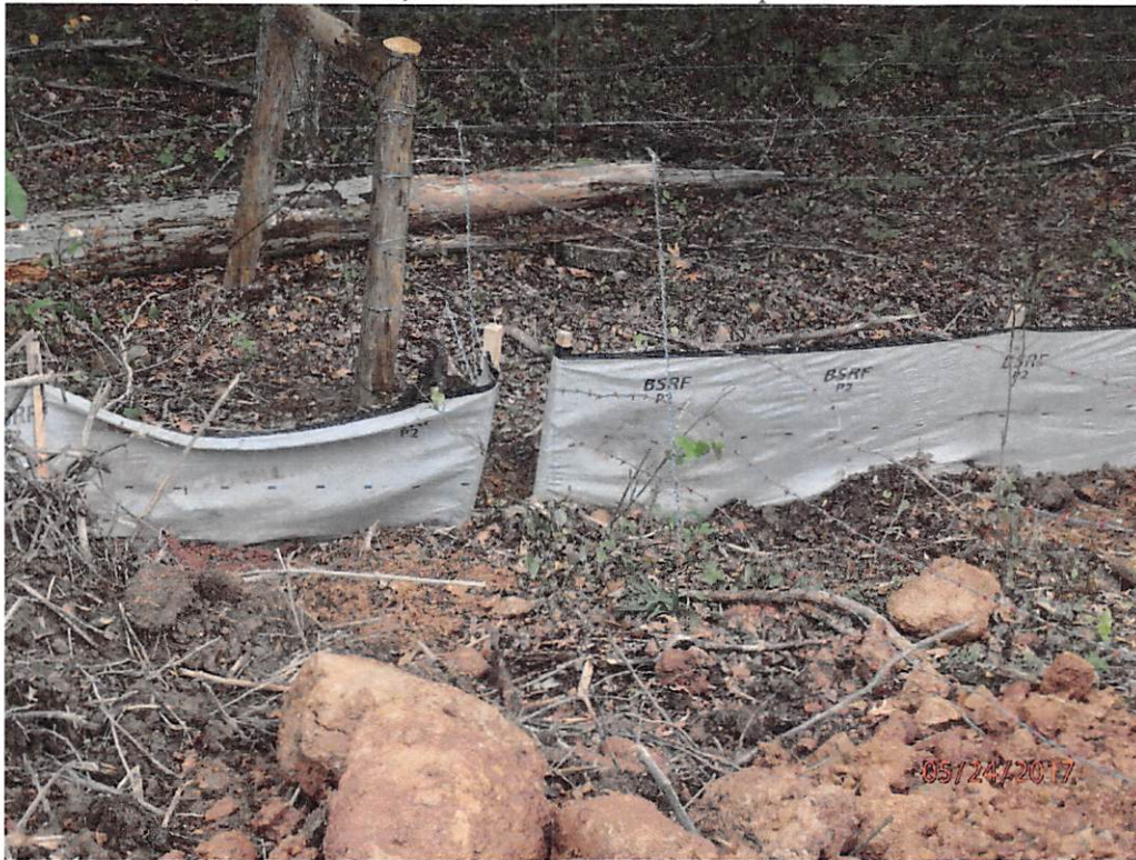
Improperly installed controls on Sherwood Lateral pipeline.
