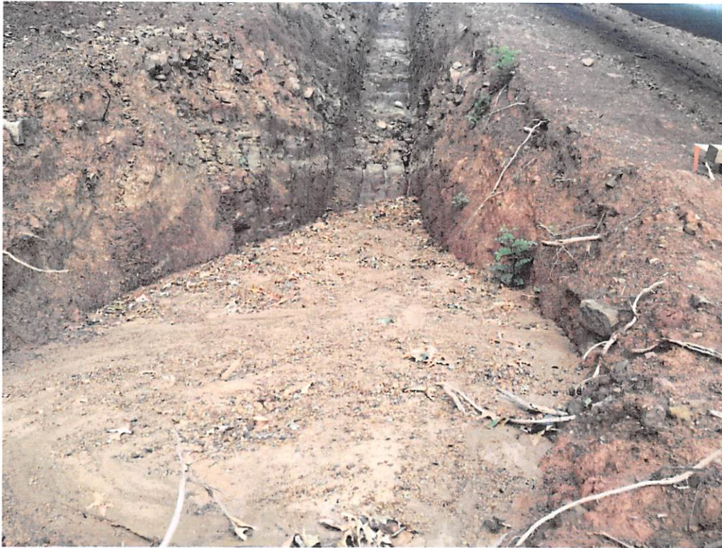
Sediment build-up at base of pipe trench.
