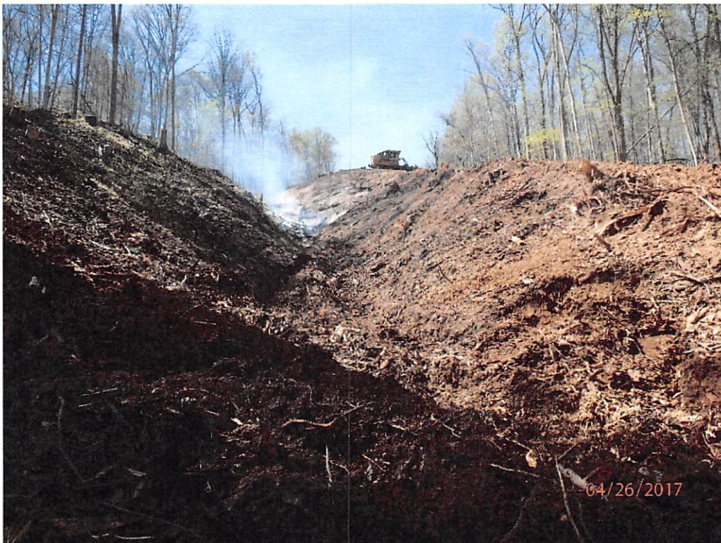
Ephemeral stream that has had equipment in channel. Soil has been disturbed with no E&S controls in place.
