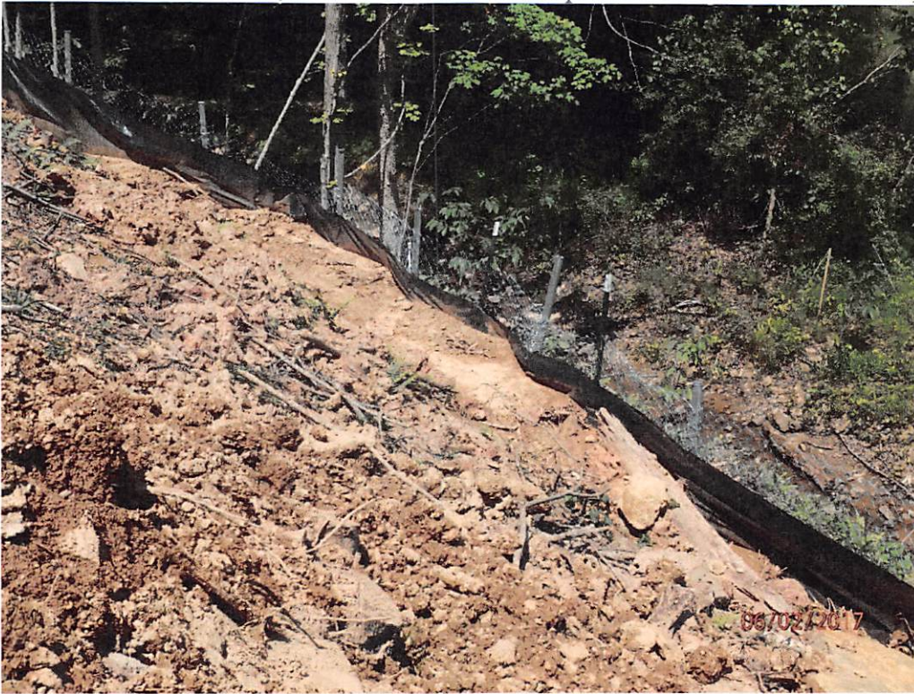
Silt fence in need of maintenance near UNT of Morgans Run.
