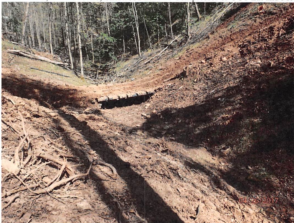
UNT of Buckeye Creek (Sherwood Lateral Pipeline ROW). Disturbed soil with no controls in place and sediment deposits in stream.
