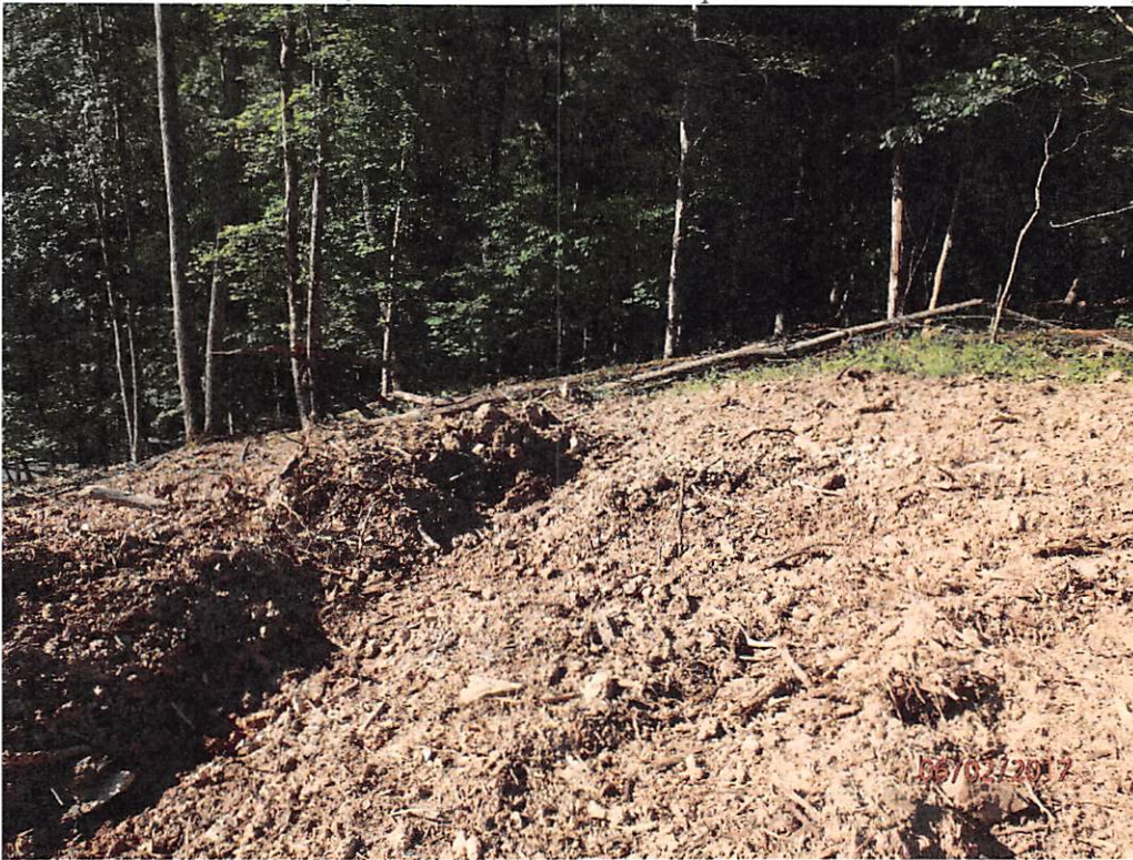
Water bars with no treatment at outlets.
