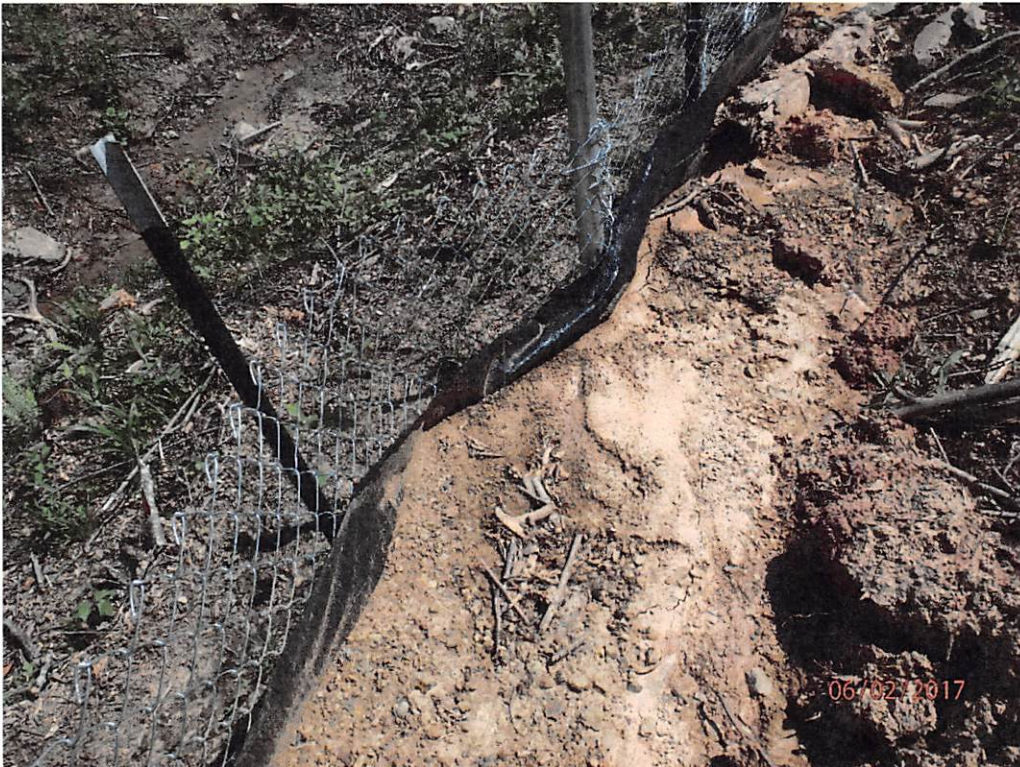
Silt fence in need of maintenance near UNT of Morgans Run.
