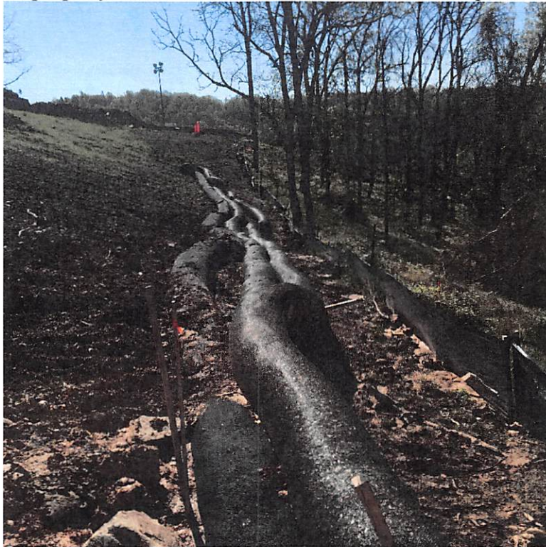
Maintenance issues and improperly installed controls (spacing and method of staking of filter sock) at Sherwood Compressor.
