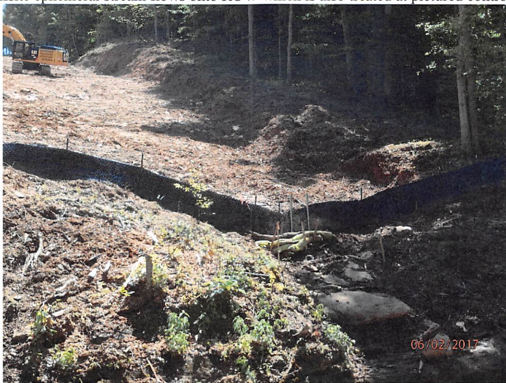
Pipeline section to the east of Englands Run where water bars were installed improperly which caused concentrated flow to be treated by sheet flow BMP's at the bottom of the hill near the receiving stream. An offsite ephemeral stream flows onto ROW which is also treated at pictured controls.
