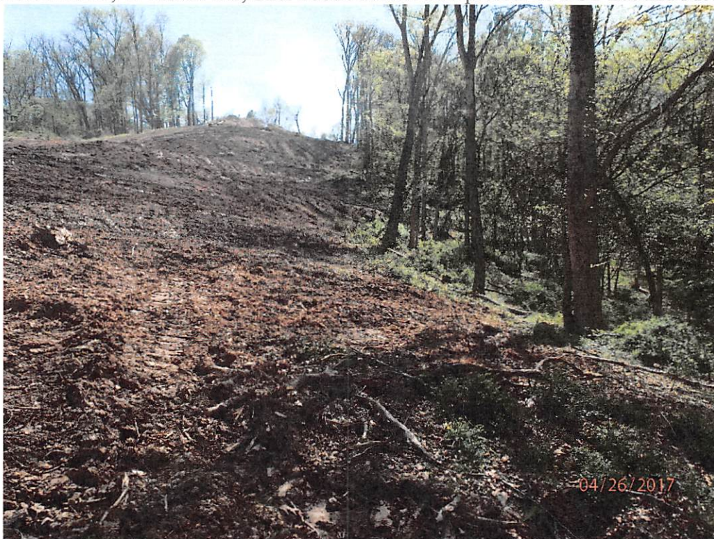
Areas of disturbed soil lacking E&S controls on Sherwood Lateral pipeline ROW.
