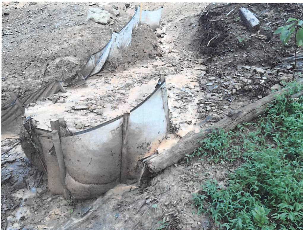
Sheet flow BMPs in need of maintenance and being used in concentrated flow areas near UNT of Buckeye Creek
