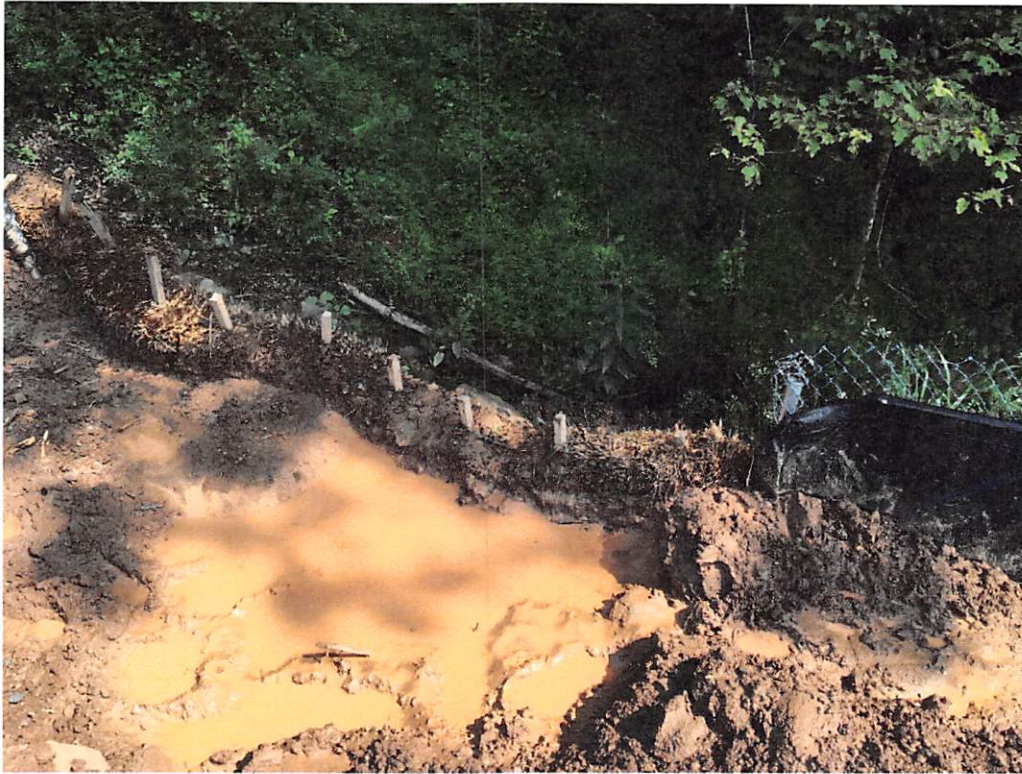
Insufficient BMPs causing conditions not allowable in UNT of Morgan's Run
