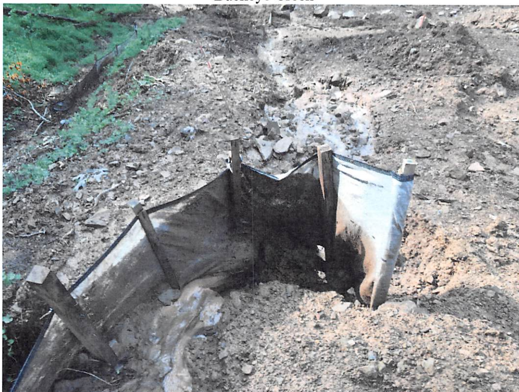
Sheet flow BMPs in need of maintenance and being used in concentrated flow areas near UNT of Buckeye Creek.
