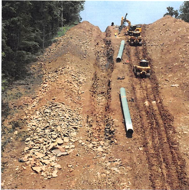
Area near England's Run where water is not being diverted off of ROW with effective water bars.
