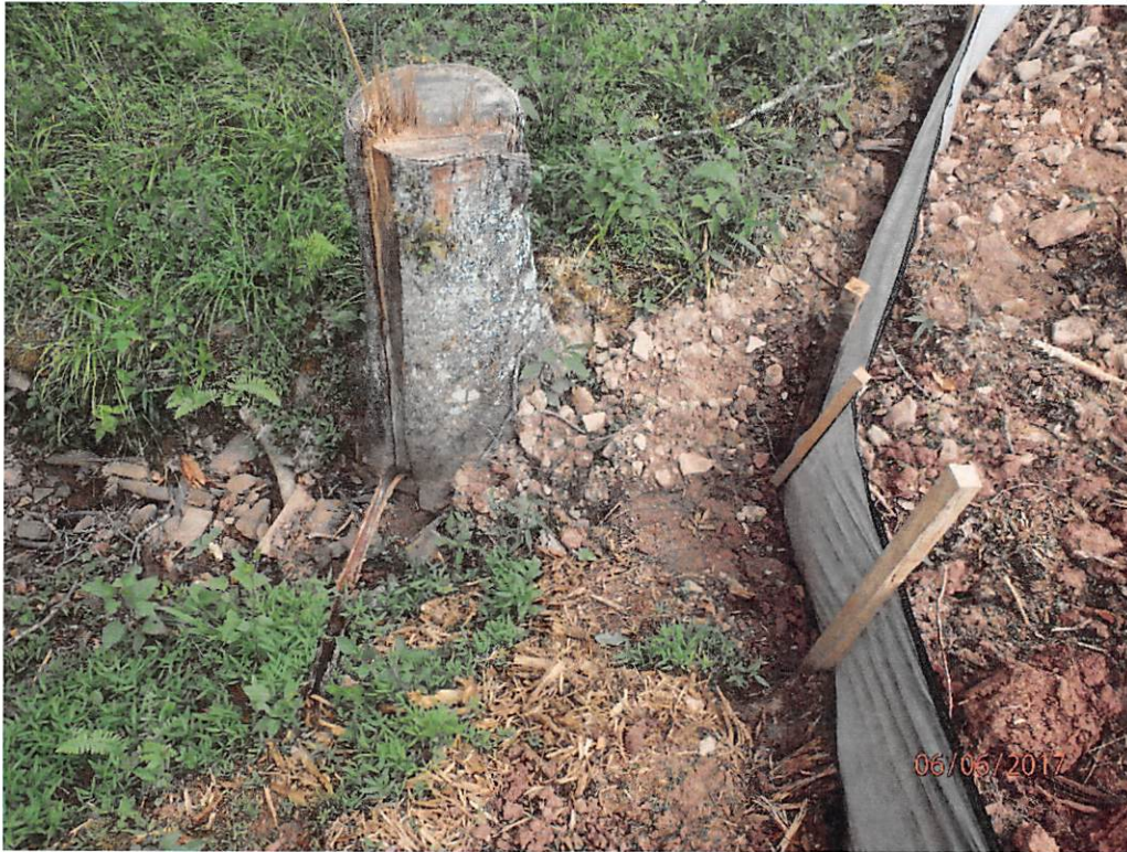
Ephemeral UNT of Nutter Fork with sediment deposits. Sheet flow BMP being used in concentrated flow.
