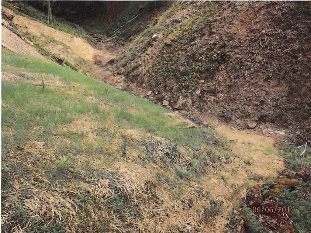
UNT of Nutter Fork with sediment deposits. Controls not in place as indicated in SWPPP.
