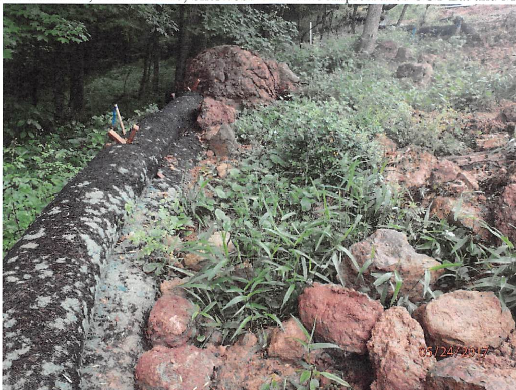
Perimeter controls below access road on compressor site.
