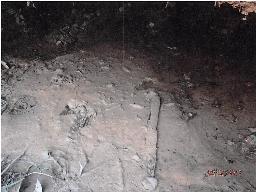
Sediment deposits in UNT of Morgans Run as a result of improper bridge installation and controls being overwhelmed due to improper water bar installation.
