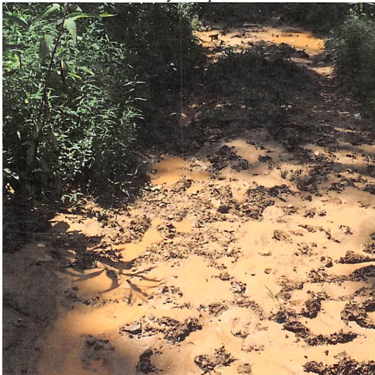
Sediment laden water leaving the site and migrating toward receiving stream adjacent to UNT of Jockey Camp Run.
