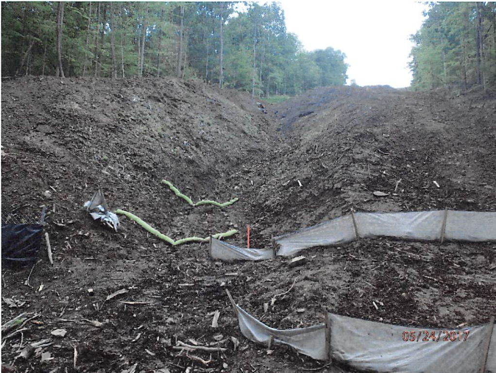
Overview of pipeline stream crossing of UNT of Buckeye Creek. Sheet flow controls being used in concentrated flow of ephemeral stream causing sediment deposits in stream. Silt fence being utilized in place of super silt fence.
