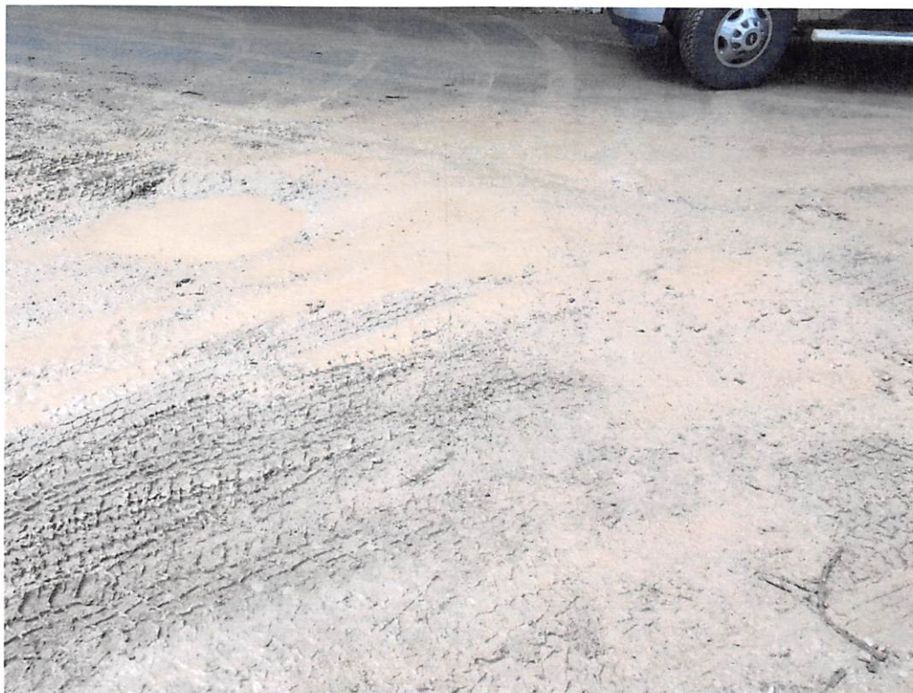
Unstable construction entrance causing mud to be tracked out onto Morgan's Run Road
