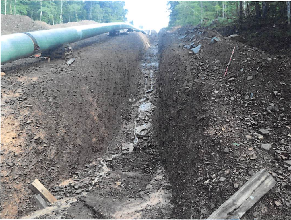
ROW with pipe trench near UNT of Buckeye creek. Water bars not in place and functioning as indicated in SWPPP.
