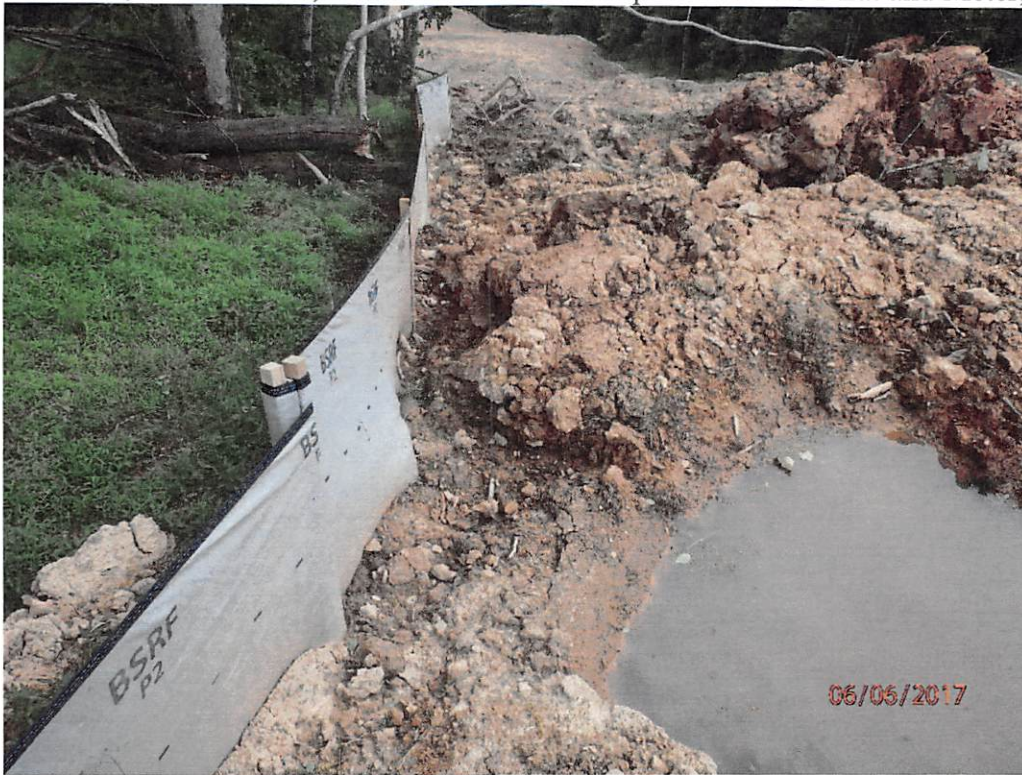
Concentrated flow from water bar that is following silt fence trench to the bottom of the hill near UNT Nutter Fork.
