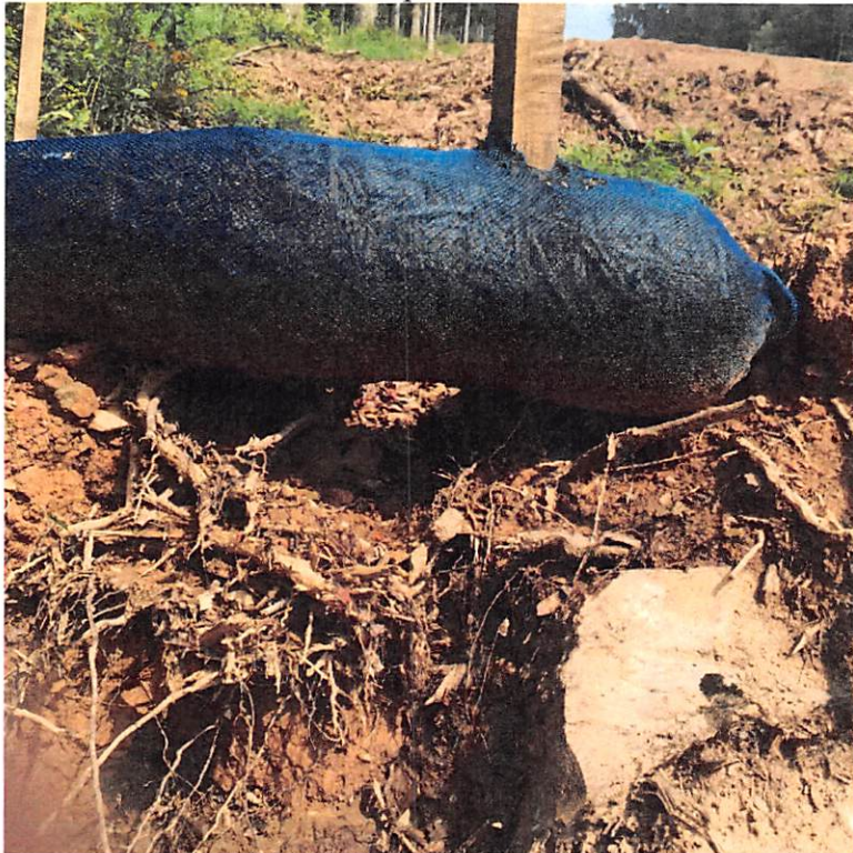
BMPs at water bar outlet near Camp Mistake Run in need of maintenance.
