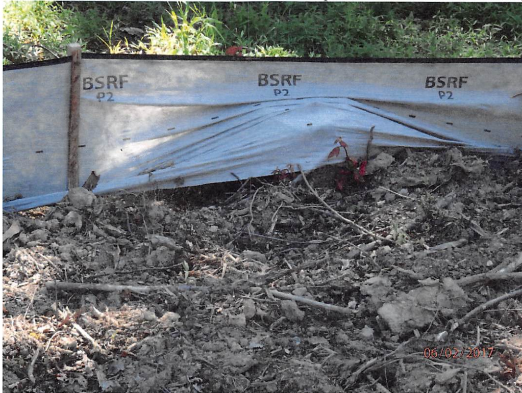
Improperly installed controls.
