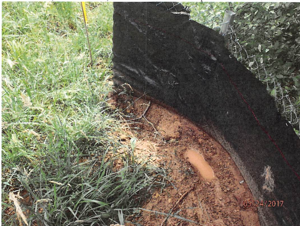
Perimeter controls west of compressor station in need of maintenance.
