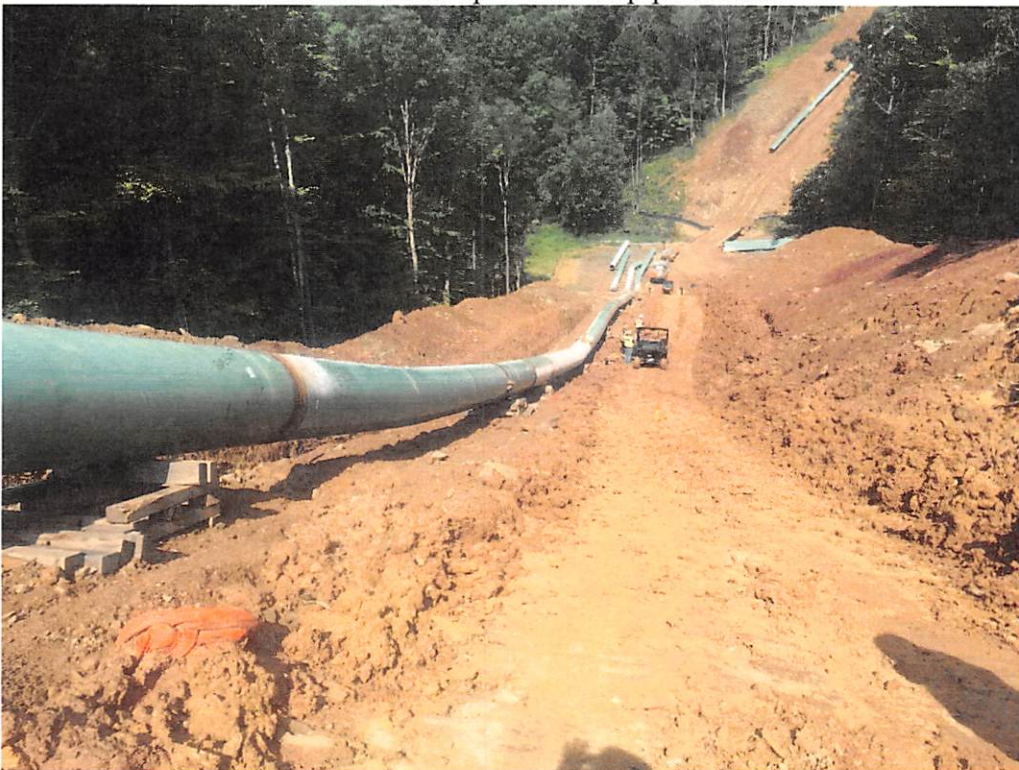
ROW near Morgan's Run showing lack of effective water bars, which caused storm water to follow pipe trench / ROW to the base of the hill.
