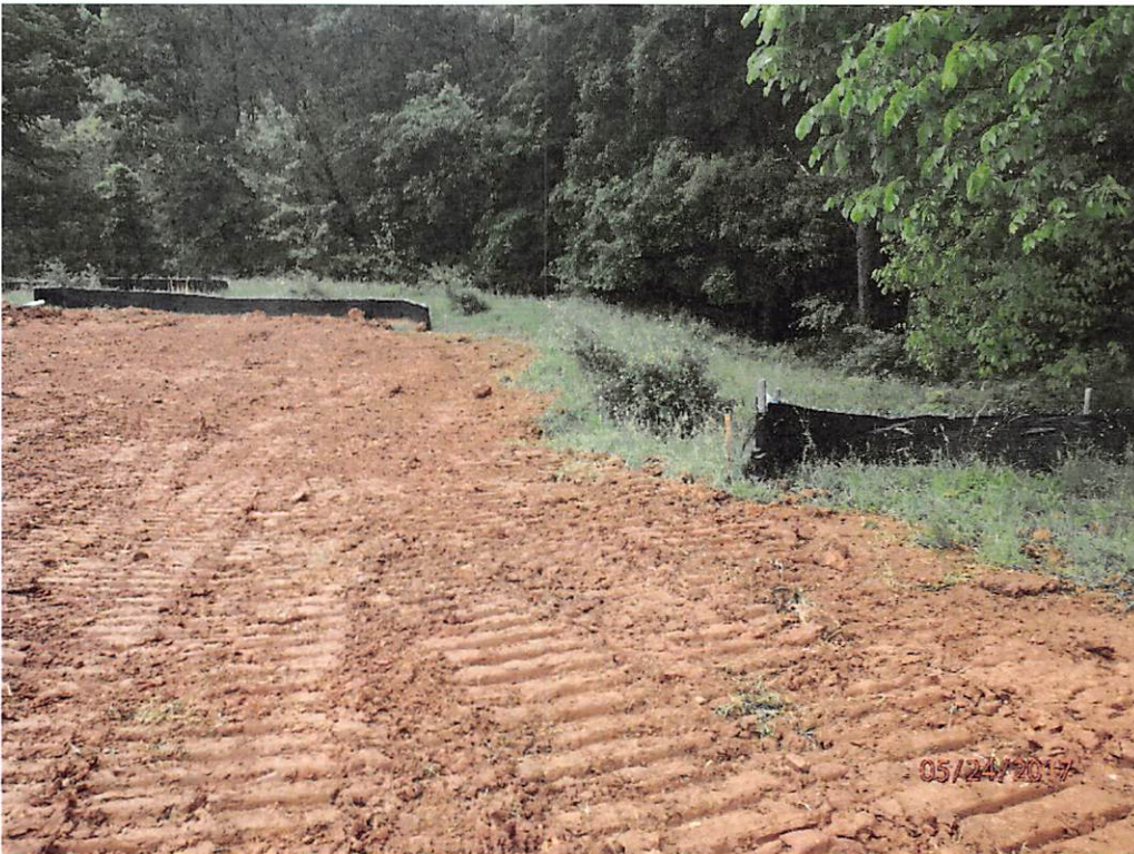
Silt fence on the western perimeter of the compressor site that needs to be extended.
