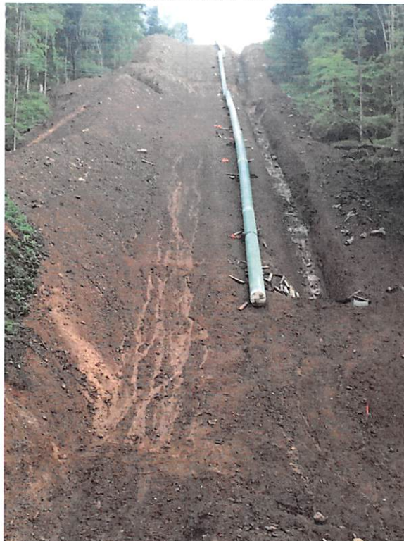
ROW with pipe trench near UNT of Buckeye creek. Water bars not in place and functioning as indicated in SWPPP.
