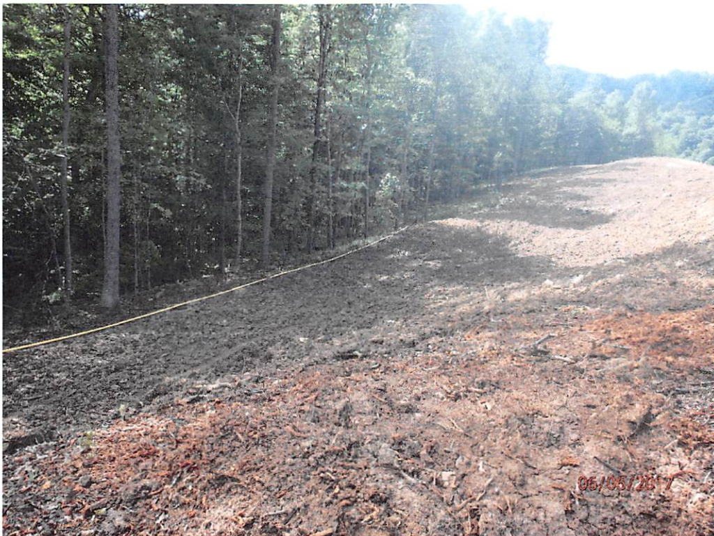
Areas of pipeline with no controls in place.
