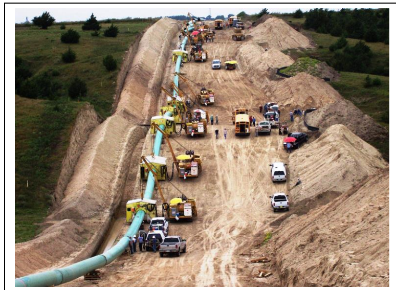
Figure 1.1.1 – Leveled work corridor for pipeline installation, showing cut hillsides and evident dewatering into the pipeline trench. Heavy equipment and pick-up trucks provide a scale
