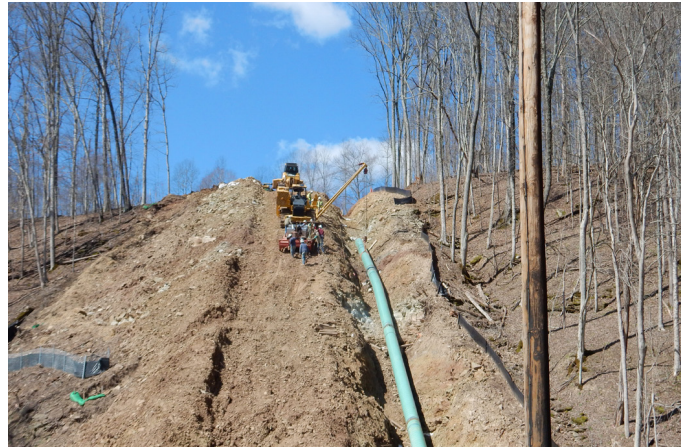
CONSTRUCTION OF OHIO VALLEY CONNECTOR: A 30 INCH NATURAL GAS PIPELINE IN WETZEL COUNTY
