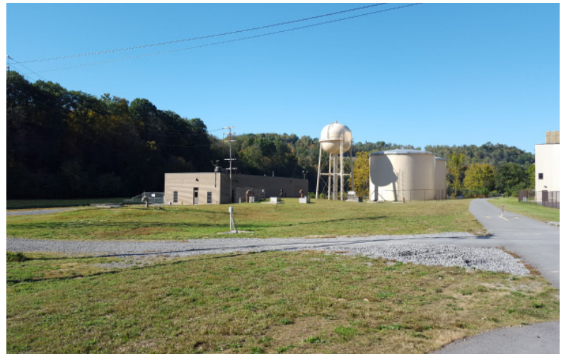
Water treatment facilities
